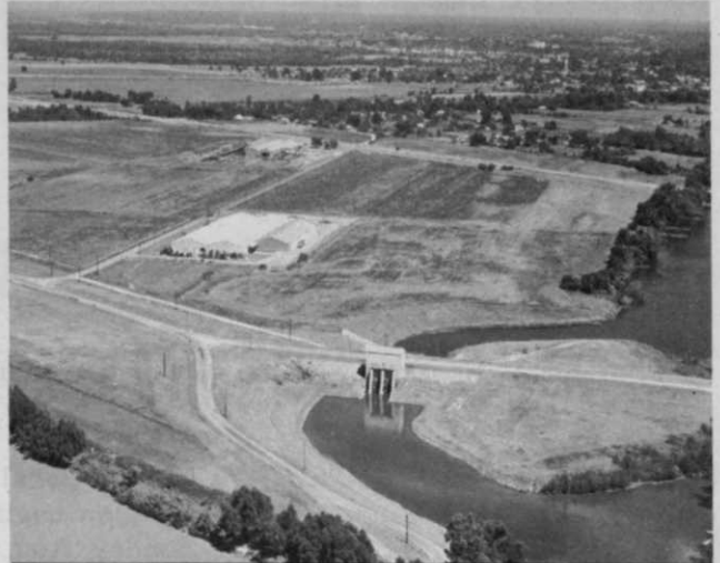
Flood gate and pumping plant at Yazoo City remove collection of interior drainage.
