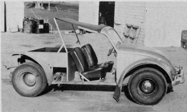
Turf buggy built from a used Volkswagen is used by Green Valley Turf Company to ride herd on the extensive irrigation system. Buggy can pass over aluminum pipe without damage, and at the same time eliminates compaction of new sod.
