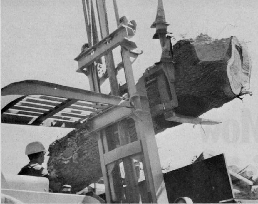
Large trunk sections are positioned by Hyster forklift and sawed to size before loading on flatbed truck for removal. All removal sites are left clean by tree crew.
