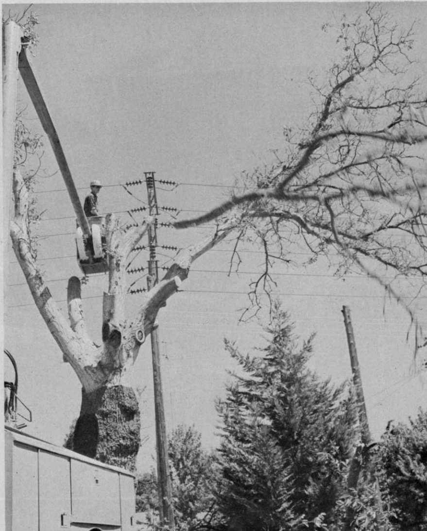
Operator controlled Sky Ranger aerial bucket is maneuvered by trimmer as he drops large limbs with aid of hydraulic pruners, rope, and self-contained chain saw. Tree foreman Ray Pifferini believed that this tree died because of excess water. Removal was delayed until tree division was sure that tree was dead.
