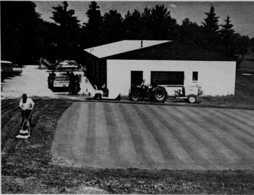
New maintenance building does much for employe morale. Building has locker room, lunch area, and storage for equipment and maintenance tools. It also houses the office of Heiss.
