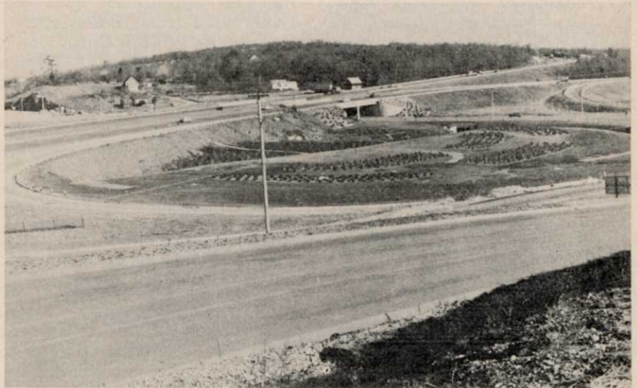
Example of formal planting in the Massachusetts program is this interchange located at intersection of Routes 128 and 37 near Braintree. Joseph L. Beasley, Department of Public Works, reports that bridge abutments, including bed plantings and individual trees are mulched with 3 inches of wood chips.
