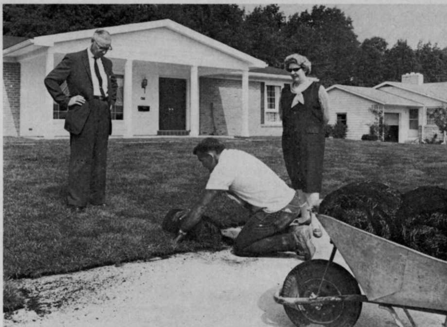
Mr. and Mrs. Wyn Behrens, publisher and editor respectively of the Marysville Journal-Tribune, appear a bit pensive as they watch sod for the lawn of their new home being laid on a 4-inch concrete base. One neighbor, watching the concrete being poured, thought the Behrens' were making a parking lot.
