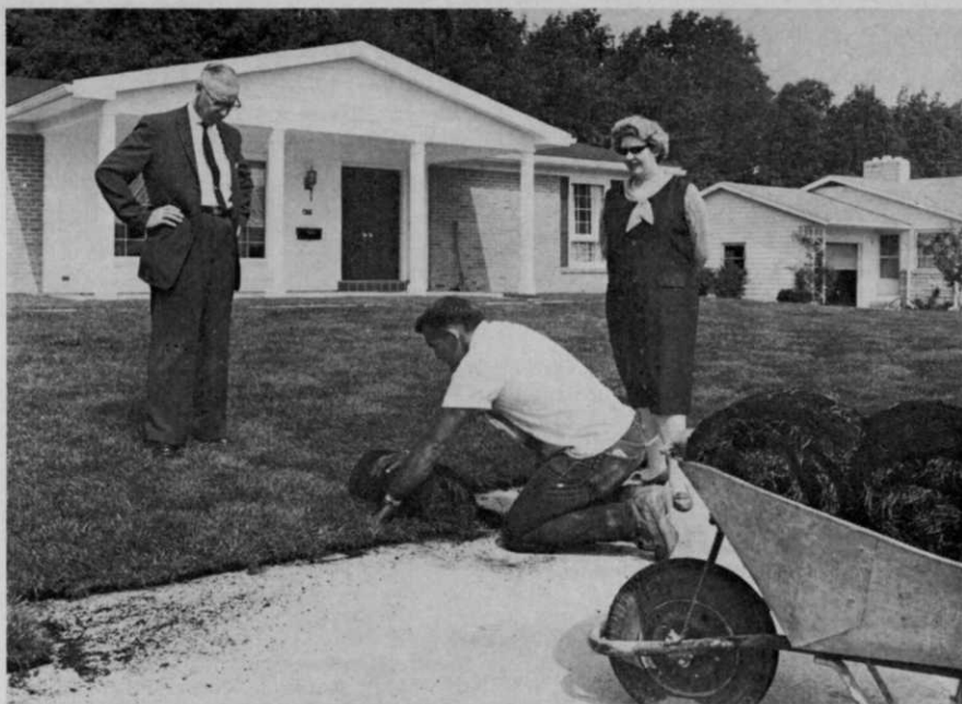
Mr. and Mrs. Wyn Behrens, publisher and editor respectively of the Marysville Journal-Tribune, appear a bit pensive as they watch sod for the lawn of their new home being laid on a 4-inch concrete base. One neighbor, watching the concrete being poured, thought the Behrens' were making a parking lot.
