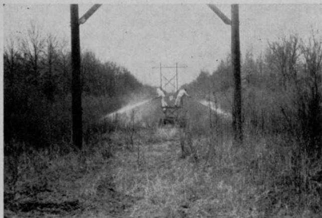
Dormant broadcast spray has been used on practically all distribution lines. Union Electric Company crew above sprays right-of-way.
