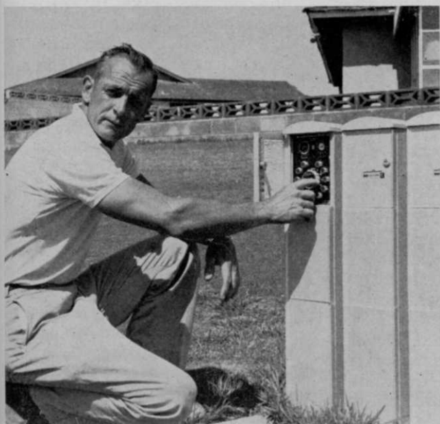
Control box for automatic irrigation system permits control of water applications with a minimum expenditure of time. Conservation of water and higher quality turfgrass are additional benefits cited for automatic irrigation systems.
