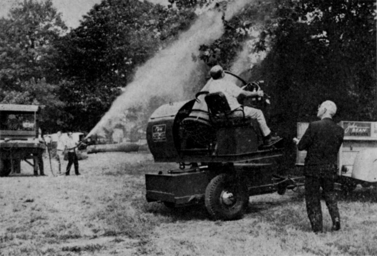
John Bean's power spraying division exhibited the Model 100G Rotomist for shade tree, sanitation, mosquito control and leaf windrowing along with one of their truck mounted heavy duty sprayers. On Rotomist is A. O. Kalp, Middletown, N.Y.
