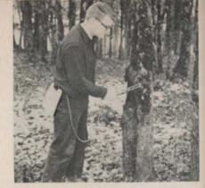
Chemical reservoir is worn at waste level and a pump supplies a constant even flow of liquid to the hatchet's check valve system. This worker is injecting a modern chemical which minimizes sprouting.
