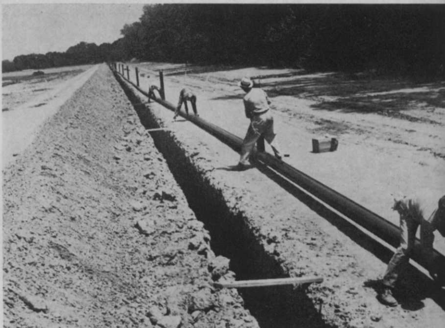
Workmen prepare to lower a section of eight-inch aluminum water main, which is part of Summit Hall's permanent irrigation system. When completed, the system will be one of the largest of its kind in the country.
