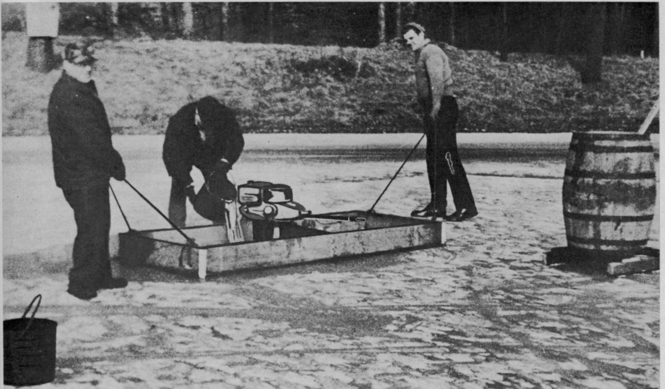
Employees of the Water Division, Massachusetts Metropolitan District Commission, treat for algae under ice. Copper sulfate solution is poured through hole in ice into current generated by outboard propeller. Rotating the complete frame 360°, effectively dispenses the algacide in an area 100' to 150' in diameter. With such a rig a reservoir of 50 to 80 acres can be treated in a minimum of time. Barrel on right holds algacide.
