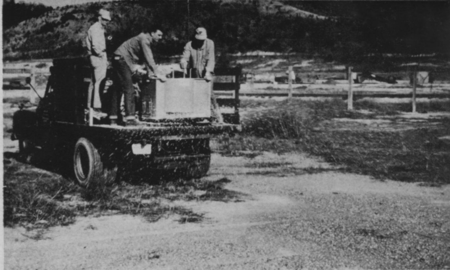
Soil sterilants are applied around steam and hydro plants by a mechanical spreader such as the one that is here operated by TVA crewmen.
