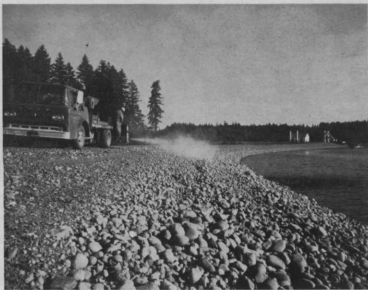
This blower dispenses copper sulfate for the Helix Irrigation District of La Mesa, California.
