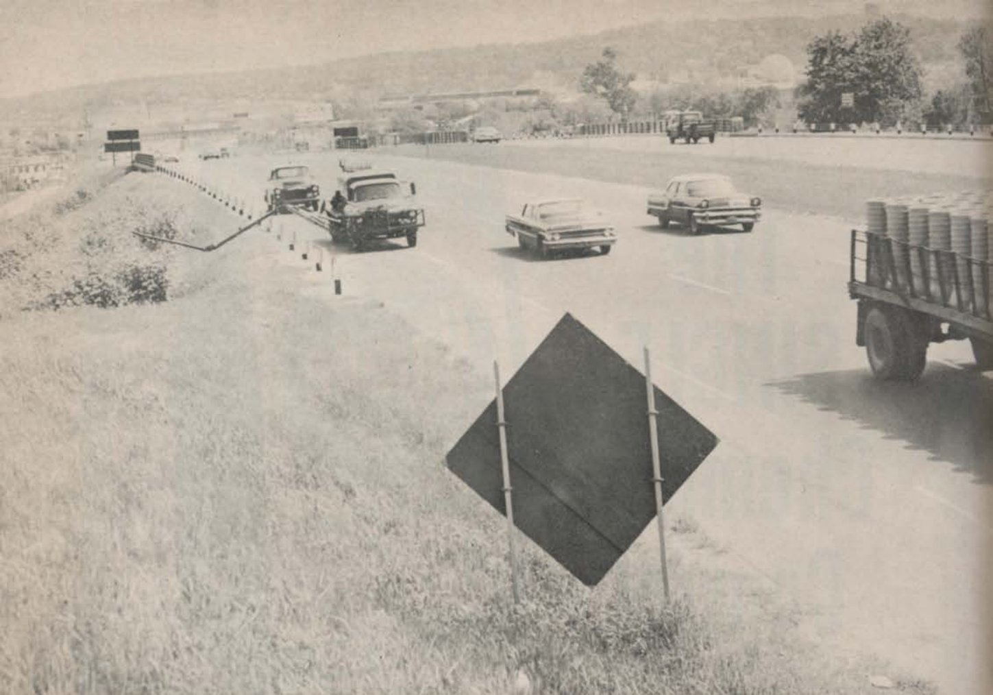
Specially adapted booms like the one in top left portion of picture help highway supervisors and contract applicators apply rights-of-way herbicides.
