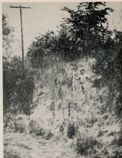
Dead brush along roads for as long as three years (as is the case here) causes public resentment. Man in background is holding a six-foot-high marker.
