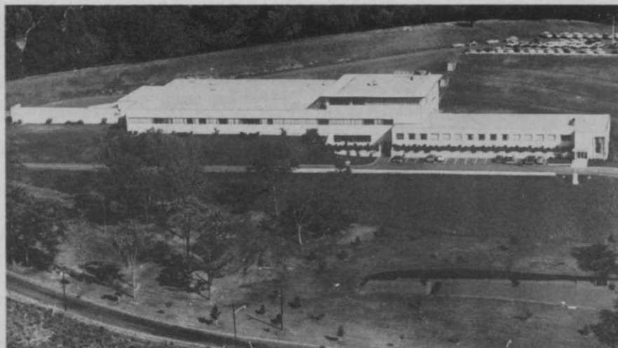
Aerial view shows the effect of good landscaping around Organon Pharmaceutical Laboratories, West Orange, N. J. Trees, turf and pond create a favorable impression to visitors and make the factory a good neighbor in this community.
