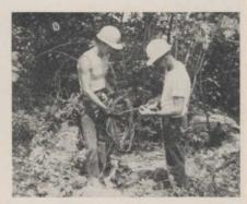
When working on a street with a trimmer lift (above left), groundmen serve as flagmen to keep traffic moving smoothly. The trimmer is signalled when traffic approaches so he won't drop brush on passing car. On the right above, groundmen coiling rope keep a sharp eye peeled for weak spots in rope, and call the foreman for an inspection of questionable strands.
