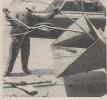
The groundman is properly attired for feeding brush into chipper. He wears helmet and goggles, stands back from hopper, and keeps his hands away from hopper by handling brush by the smaller branches. Modern chippers have every possible safety measure built into them, but the operator must nevertheless be properly attired, and follow even the most routine safety precautions.
