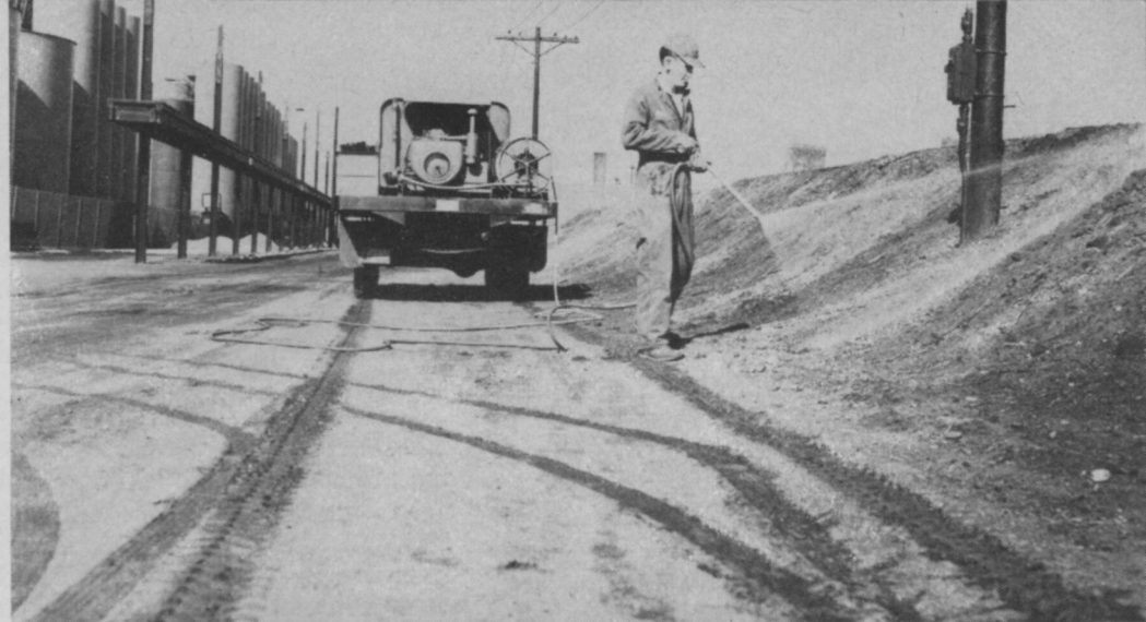
Roadways inside industrial parks must be kept weed free. This sprayman uses a truck-mounted boom for accessible, level areas; a small sprayer for the hard-to-reach slopes.
