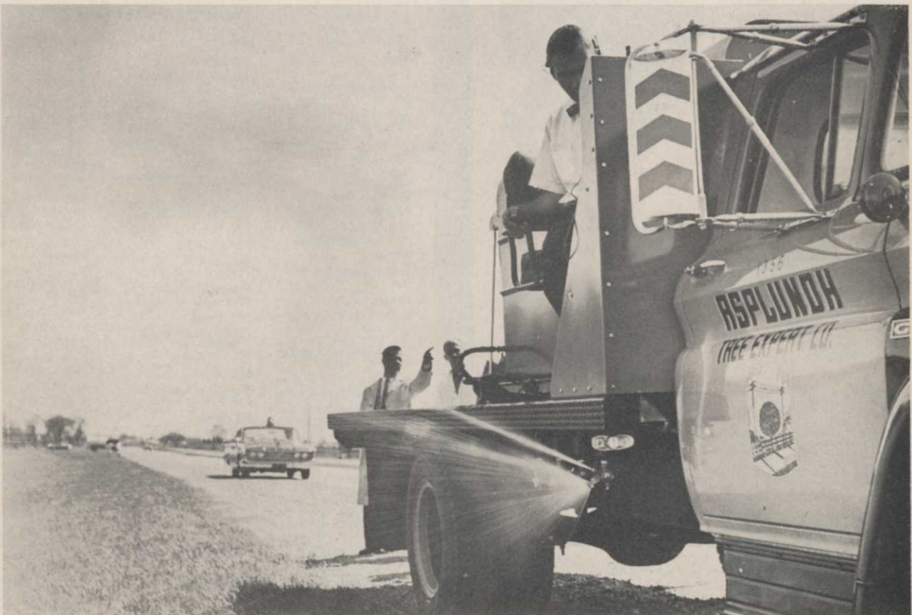
Typical contract sprayer on highway job. Asplundh had this spray rig especially built by the John Bean Division, FMC Corp.
