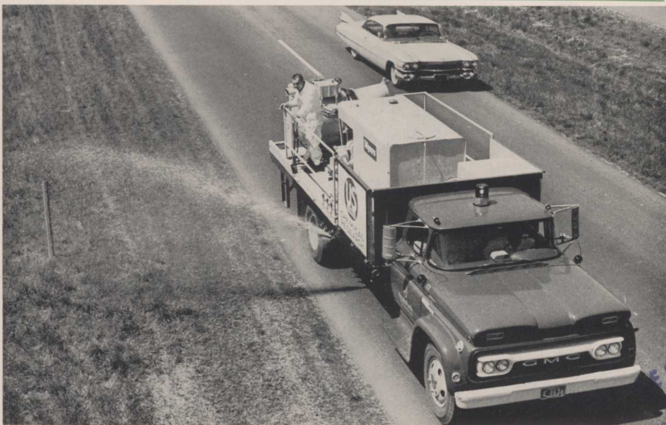
A fixed nozzle on the bed of Naugatuck's demonstration spray unit covers a 20-foot swath with a spray of MH-30, new growth retardant.
