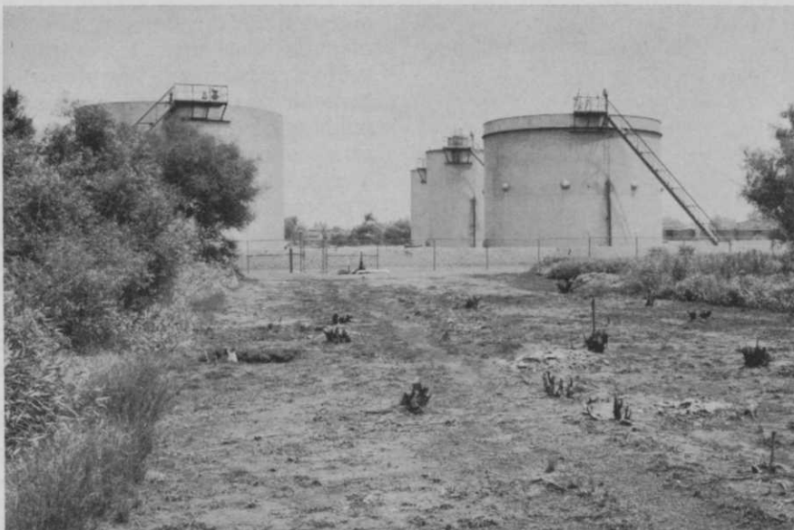
One suggested application for Chlorea herbicides is for control of weeds around tank farms and pipe lines. This installation, including the pipeline path in the foreground, was successfully treated with Chlorea, with less fire hazard and easier accessibility as direct results.
