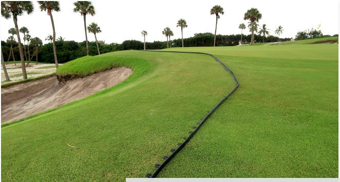
Sections of plastic landscape edging are used to divert surface water away from bunkers to minimize sand washouts.
