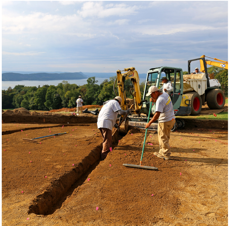
LATERAL DRAINAGE PIPES SHOULD BE SPACED NOT MORE THAN 15 FEET APART AND HAVE A CONTINUOUS SLOPE OF 0.5 PERCENT OR GREATER TO THE MAIN DRAIN LINE.
