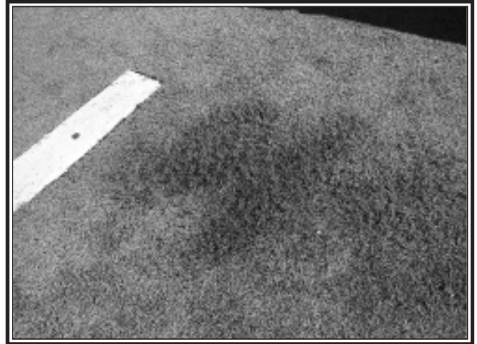
Significant fiber deterioration was evident directly in-front of the girls' softball pitching rubber.
