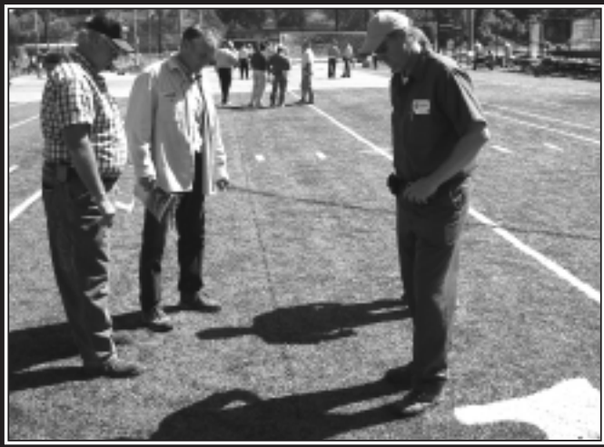
Not exactly seamless. District 4 Meeting attendees observe a large, not-easily-repairable seam in the playing surface of this synthetic infill system.
