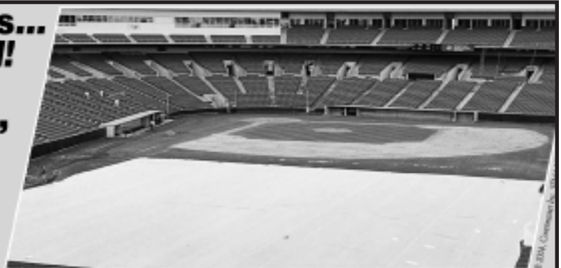
A multitude of permanently in-laid lines designating the playing areas for several sports, painted lines, and use of skin infield-colored carpet for a softball field all in one area creates a visually confusing surface.
