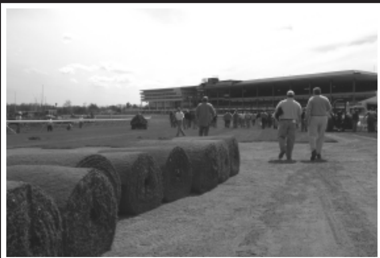
Big roll sod is lined-up to be installed on a racing chute at Monmouth Park, Oceanport, NJ. The turf course at Monmouth Park racetrack was the site of the afternoon sessions of the Spring Field Day, April 13, 2006.
