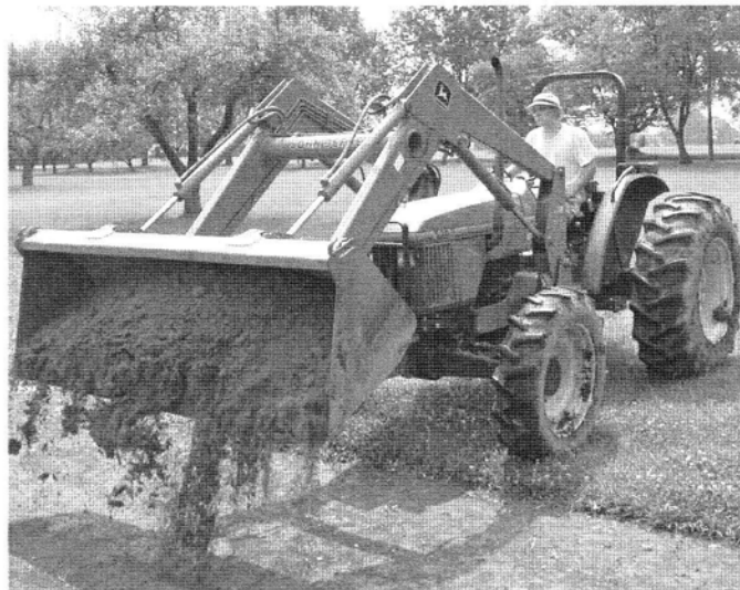
Excavated pits were filled with infield mixes using a front-end loader.
