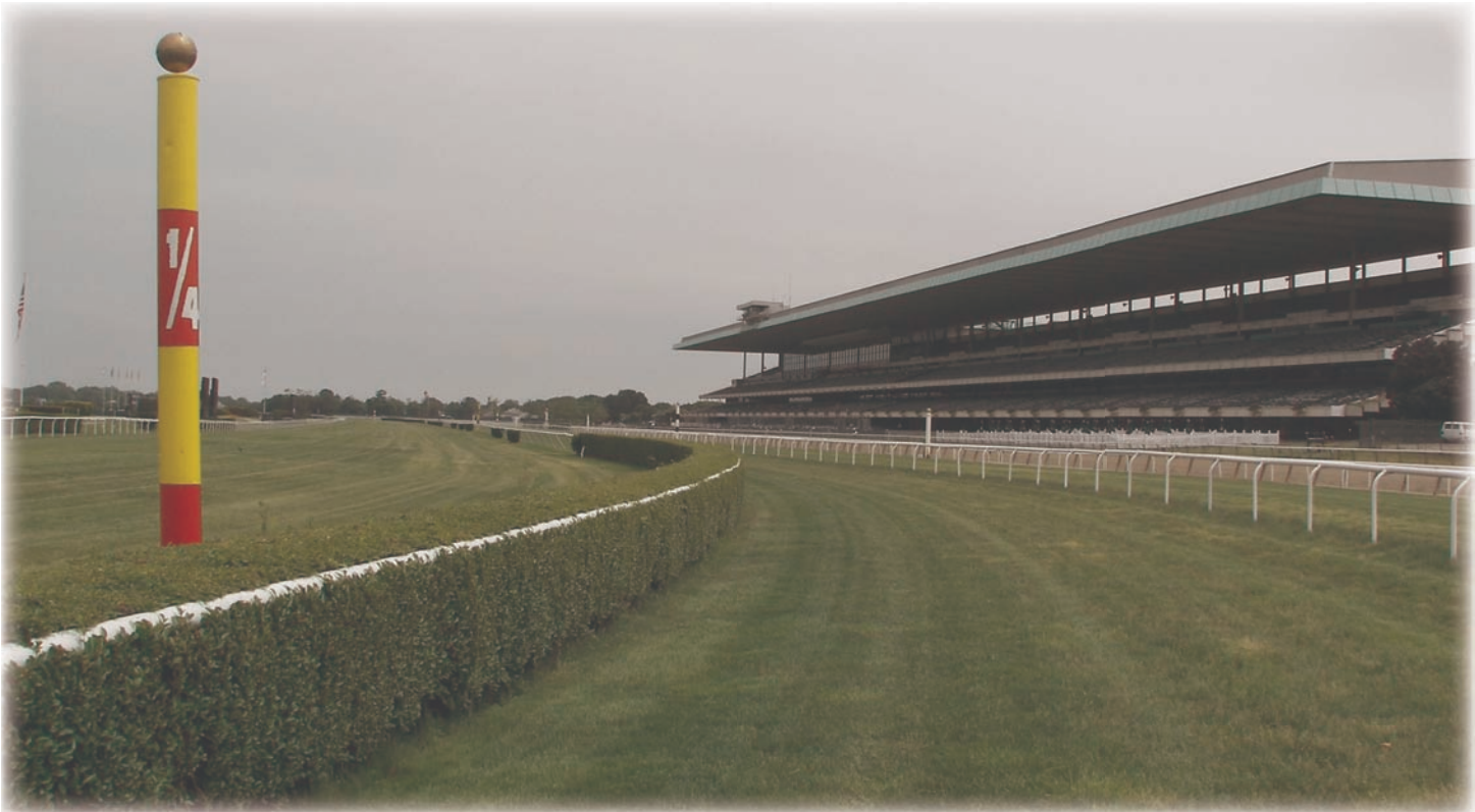
Inside (Inner; 1 \frac{3}{16} miles) and outside (Widener; 1 \frac{5}{16} miles) Turf Course at Belmont Park, Elmont, NY. Photo by Brad Park, May 2010
