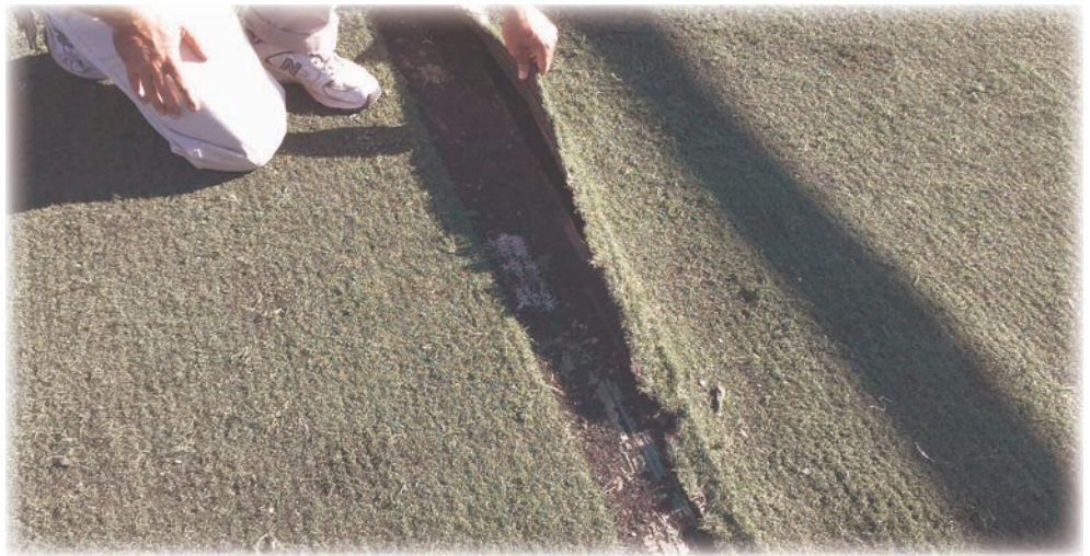
A lack of attention to synthetic fields may result in severe seam damage as in the case of this all-rubber infill synthetic field (Photo by Matt Olivi).
