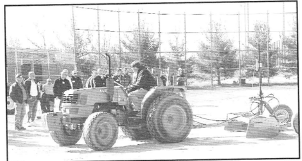
Skin surface laser grading: Sean Connell, Georgia Golf Construction
