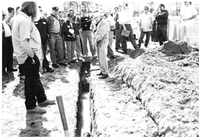
Dr. Henry Inkyk, SFMANJ Advisor and GSI Sports Field Consultant describes the steps in installing drainage.
