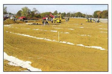
Following the 2005 Monmouth Park racing season, the inside hedge was removed, topsoil was stripped, and underdrains were installed in the subbase of the backstretch of the Monmouth Park turf course in November 2005 in preparation for the 2006 racing season and the 2007 Breeders' Cup.
