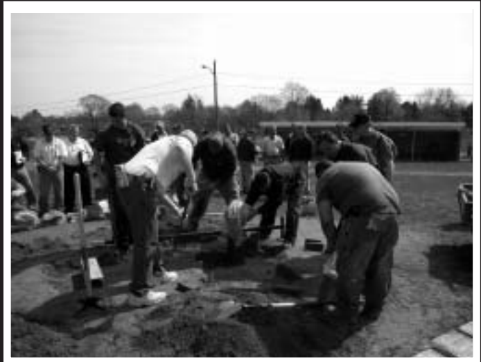
Field Day attendees were given the opportunity to build a pitcher's mound as part of the SFMANJ Spring Field Day 2006 held at Shore Regional High School, West Long Branch, NJ on April 13, 2006.
