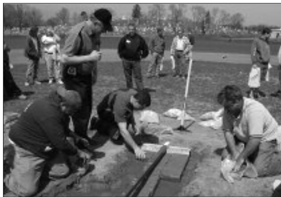
Spring Field Day attendees help to build a pitchers' mound under the guidance of Ron Martin, Mar-Co Clay Products, Inc. at Shore Regional HS.
