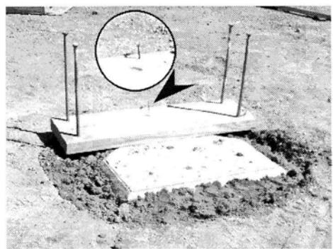
the nail. Position the board with the nail contacting the home plate at the apex and stabilize the board utilizing landscape spikes. The nail can then be used as a connecting point for your string or tape measure, which can be pulled in any direction from that point.
