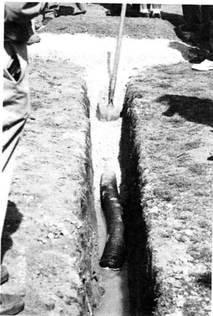
The drainage ditch closer using pea gravel and perforated pipe. The secret is not using fabric.
