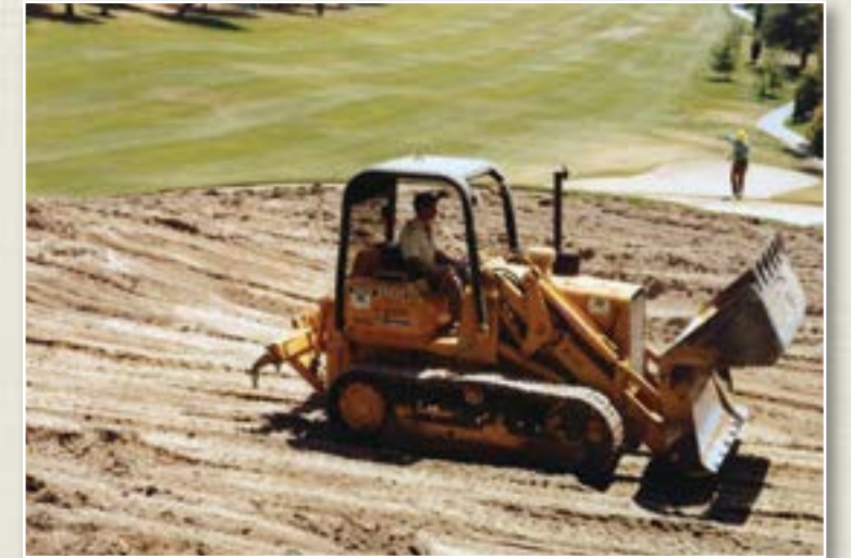
Steve on bulldozer rebuilding the #1 green at San Jose Country Club
