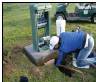
New pad and satellite ready for wire installation
