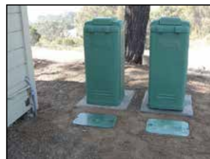
Final Product with valve boxes and splices in conduit
