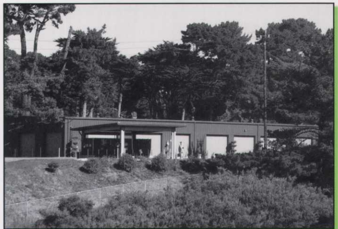
Lake Merced Golf Club Turf Facility built by DBD Structures
