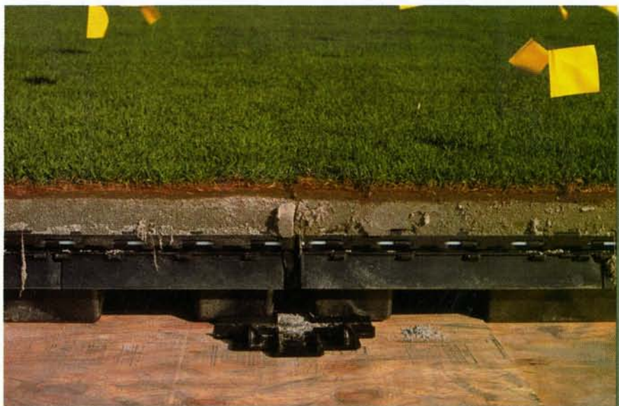
Modules are 46 in. square with channels 22 in. apart on all four sides. These channels can be sealed to create a ventilation system that can draw air down through the turf, provide oxygen to the root zone and provide drainage for irrigation and removal of carbon dioxide.
