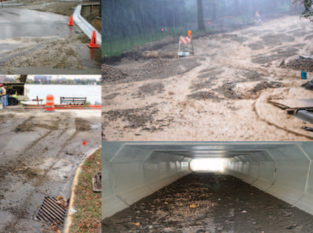
Figure 2. Everyday images of sediment losses from construction sites in urban environments. Images: contractorreport.blogspot.com
