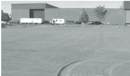
Above: All vehicle surface tracks were removed by hand to ensure a proper finished grade on the playing surface.
