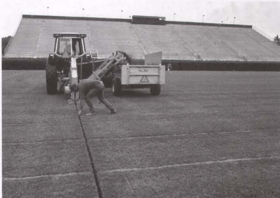
Above: Installing a grid drainage system.
