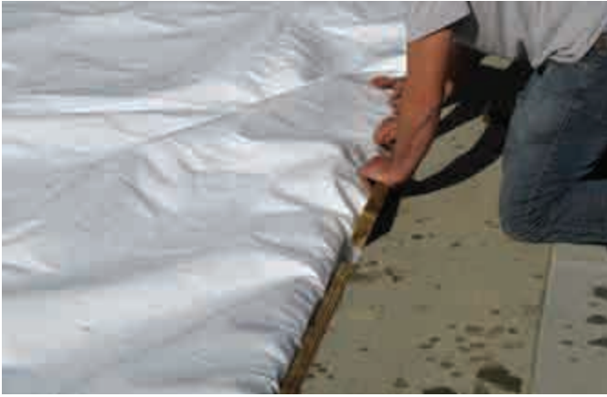
Fabric membrane being locked into anchoring system (Greenville, PA).
