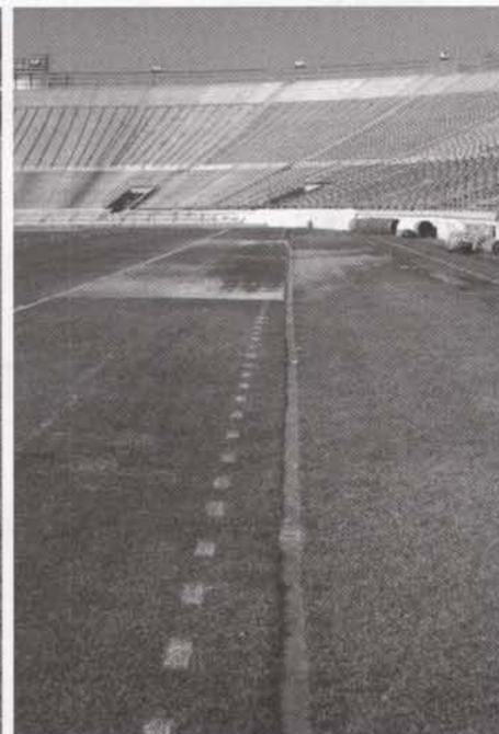
The mistake some managers make is running pipe under a native soil field and capping the last six inches of the trench with the topsoil they removed. I found many of these systems seldom conduct water through the pipes for very long. Once that surface soil becomes compacted, the water can no longer make it to the drainage pipe.
