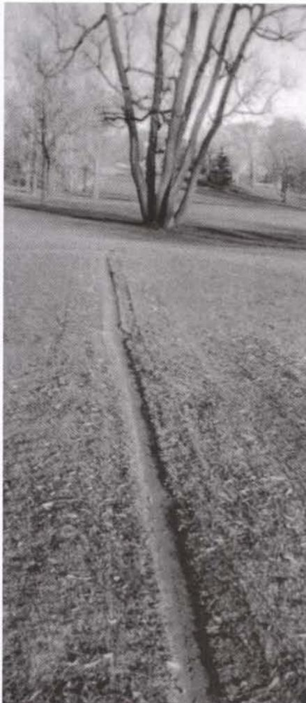
trenching is installed. To be ready for fall sports, you should put down about 3/8 inch of straight sand across the whole system in spring. Run some test strips in the field surrounds until you become calibrated. This is a lot of sand. It looks like you are burying the grass. The grass will grow through the sand and in four days you'll be mowing again so don't be too concerned. You shouldn't plan on playing on the newly topdressed turf for some time.
