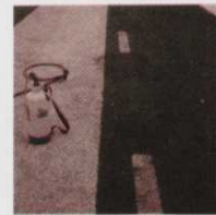
10:10 a.m. Section of Temp-Line completely removed.
