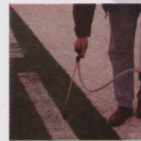
10 a.m. Pre-wet Temp-Line section and apply Temp-Line Eraser.
