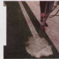
10:05 a.m. Rinse with low-pressure water.
