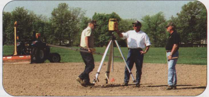
University of Missouri research associate Brad Fresenburg, right, works with Mike Munie, center and Dave Niebruegge of MJM Services to grade the new infield. Using a laser-leveling device they were able to create a .5 percent slope on four quadrants surrounding the pitcher's mound as the center point.
