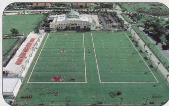
Miami Dolphins Training Facility, Professional Football Field of the Year
